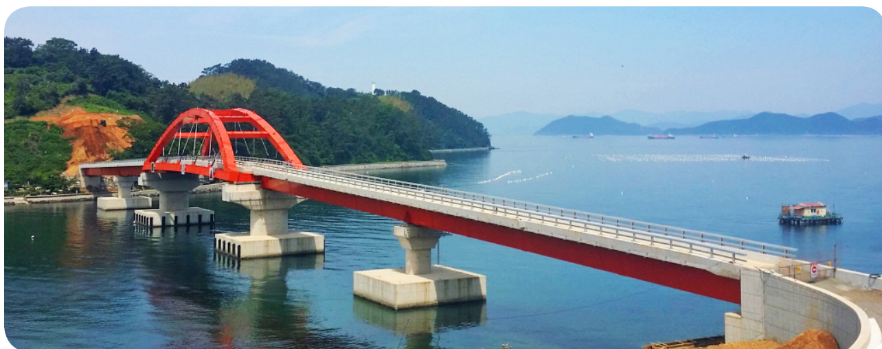
• 황덕연도교 / L=2@50m+Arch\ 60m+2@50m=260m , B=5.5m , H=2.2m
