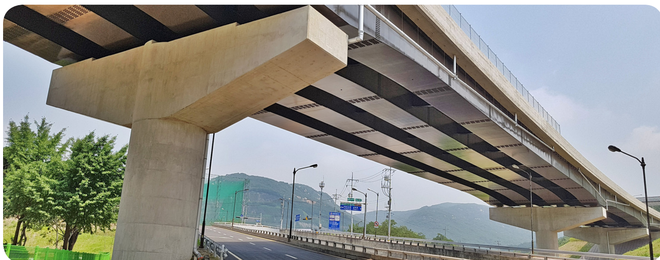
• 삼막교 / L=48m+78m+49m+30m=205m , B=24.3m , H=2.2\sim3.2m , R=1100
