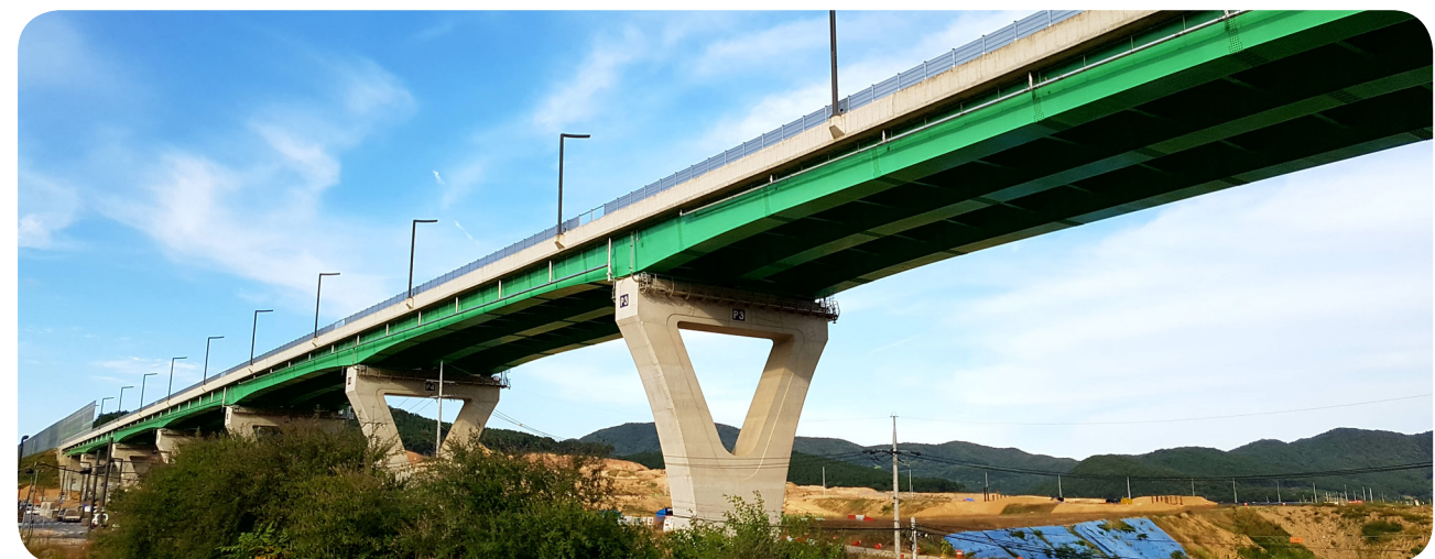
• 신리교 / L=50m+7@65m+50m=555m , B=21.2m , H=2.4\sim3.0m
