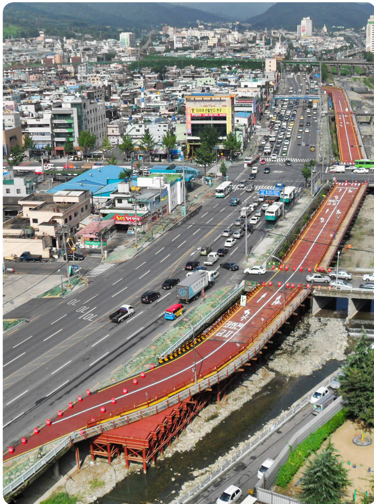
• 석전가교 / L=26m+18m+110m+11.7m+119m+83.6m+9.8m+25m+10m+18m=430m , B=8m
