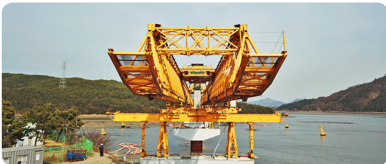
• 광영교 / L=2(3@45m)+5@50m=520m , B=13.5m , H=2.8m , Beam Weight=175ton
