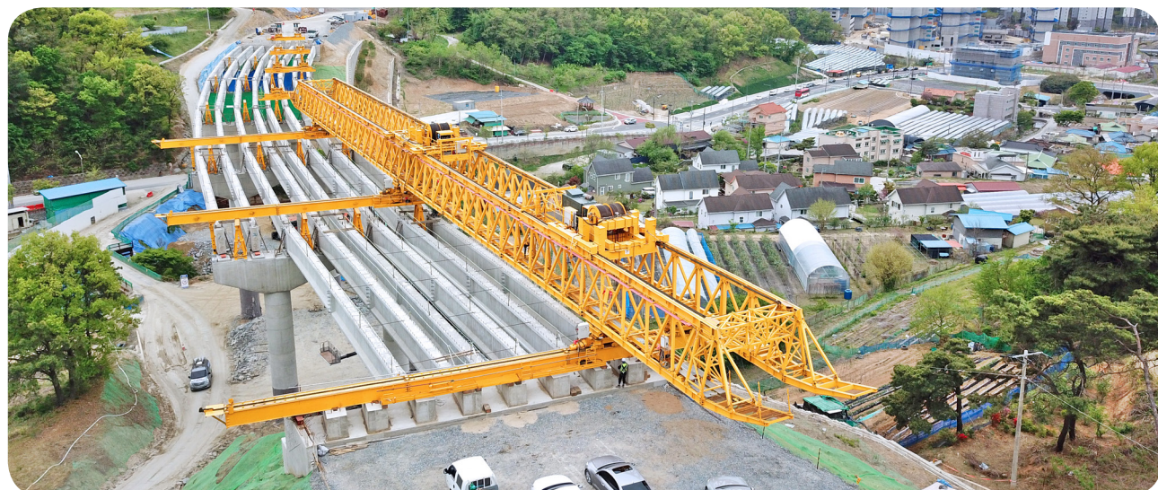
• 용정3교 / L=3@35m+3@35m=210m , B=20.9m , H=2.2m , Beam Weight=80ton
