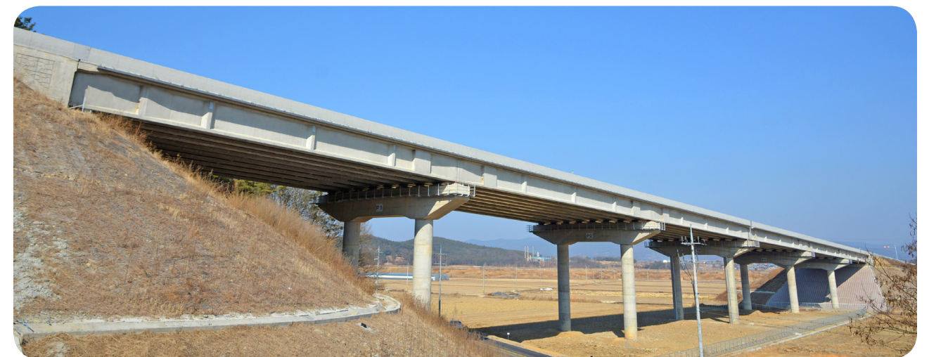
• 서제교 / L=(40m+50m+50m)+(50m+50m+40m)=280m , B=24.3m , H=2.7m
