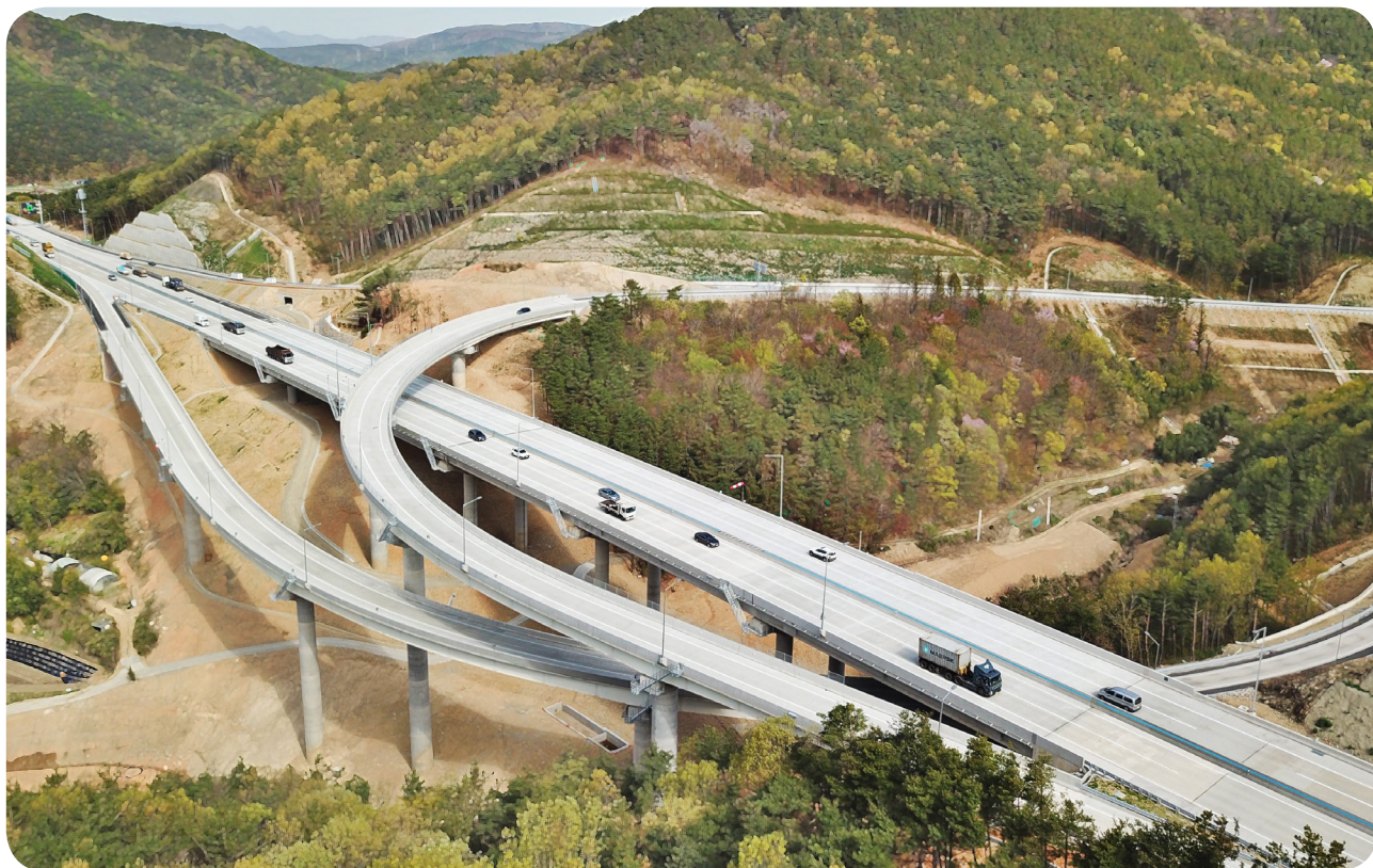
• 와여2교 / L=3@45m+3@45m=270m B=24.3m , H=2.3m
