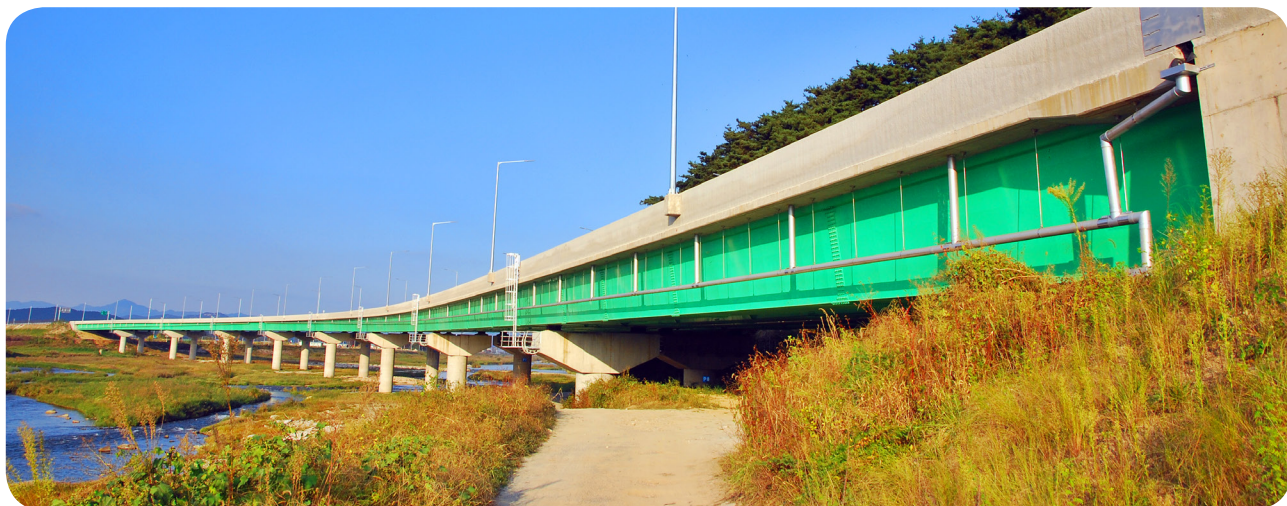
• 요천교 / L=50m+7@60m+50m=520m , B=20.9m , H=2.2m , R=680
