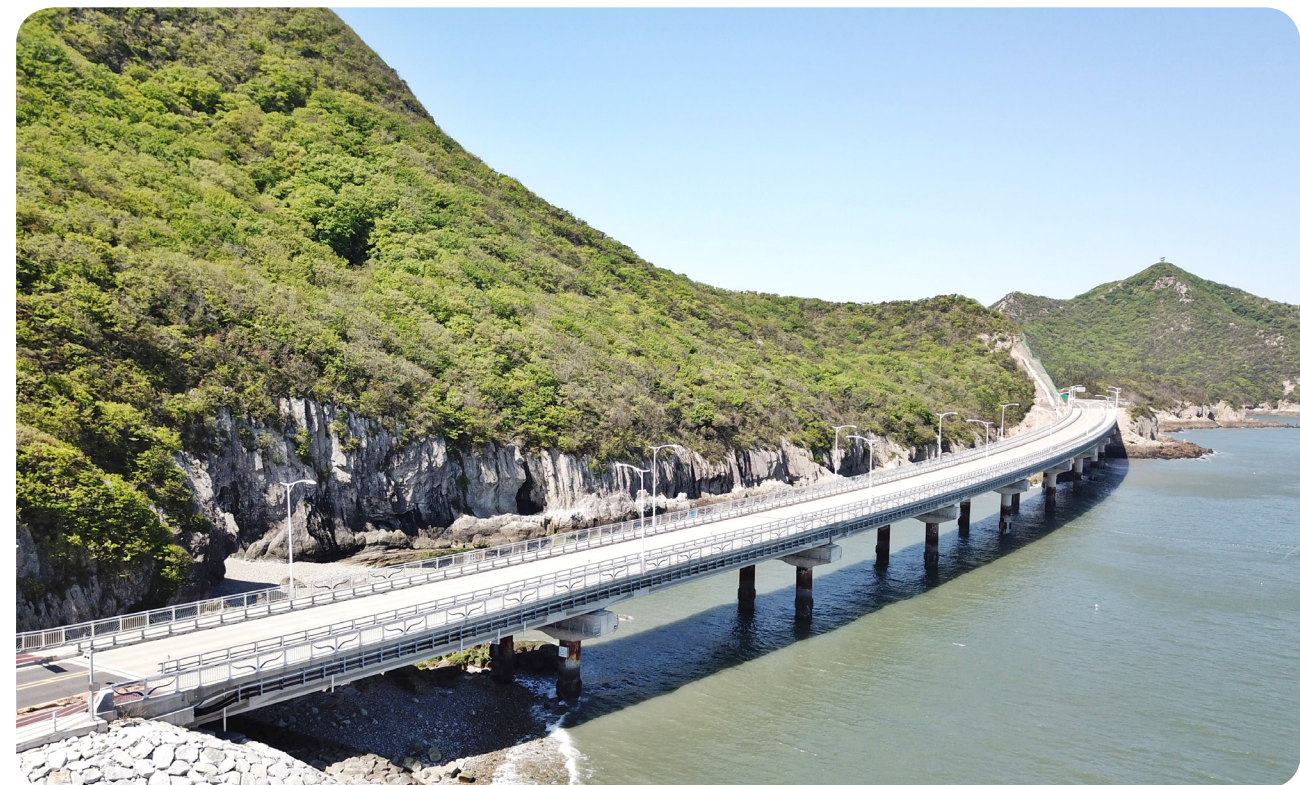
• 신시해안교 / L=40m+45m+3@45m+3@45m+45m+40m=440m , B=16.5m , H=2.3m
