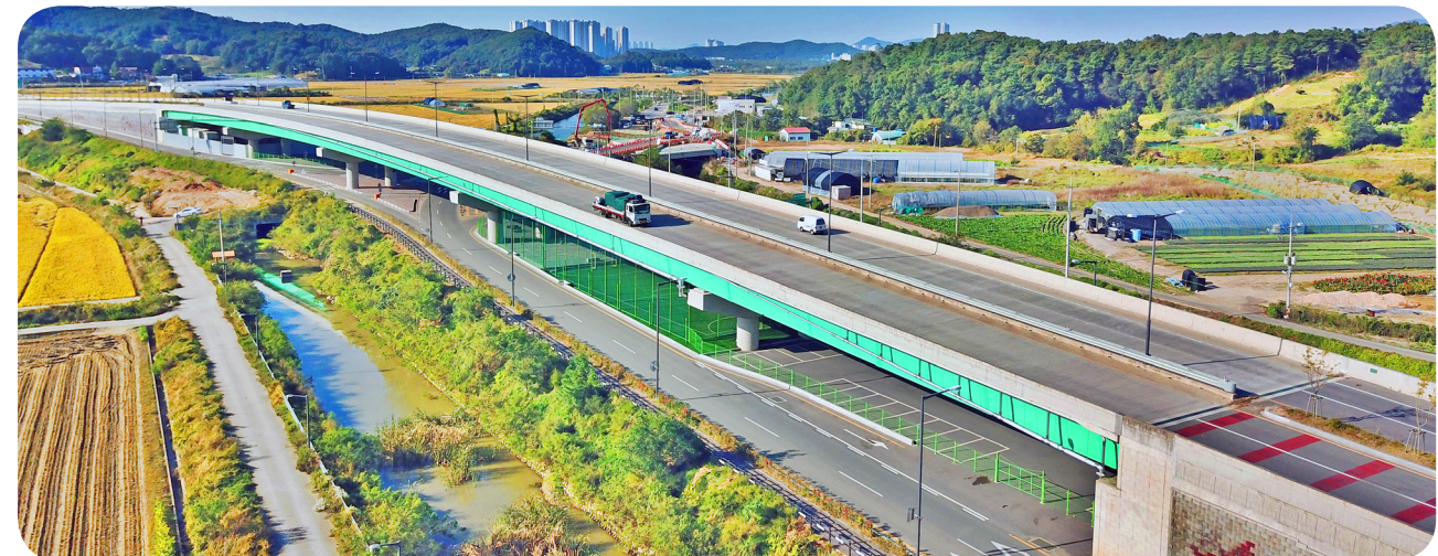
• 삼화2교 / L=50m+3@60m+50m=295m , B=22.4m , H=2.6m
