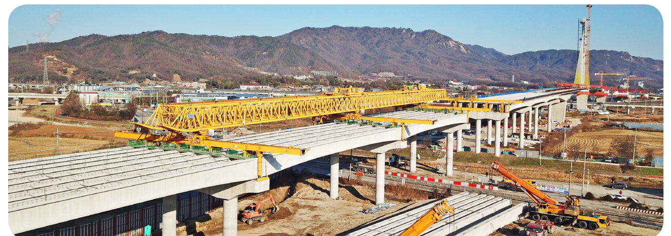
• 회암천교 / L=5@40m+3@48m+4@40m=504m , B=24.5m , Beam Weight=175ton
