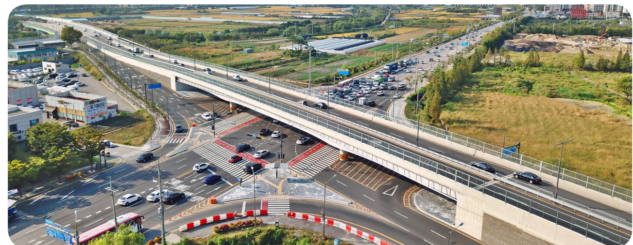
• 탐동고가교 / L=36m+60m+44m=140m , B=16.94m , H=1.8\sim2.6m
