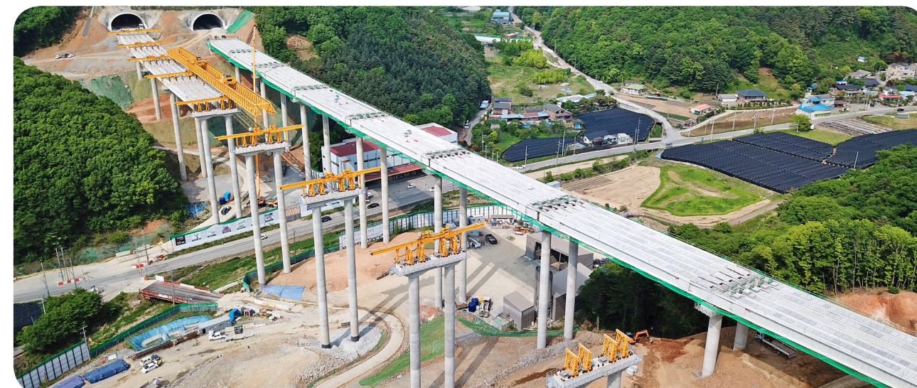
• 해곡교 / L=3@47.5m+3@50m+3@42m=418.5m , B=16.1m (편도), H=2.5m , Beam Weight=167ton
